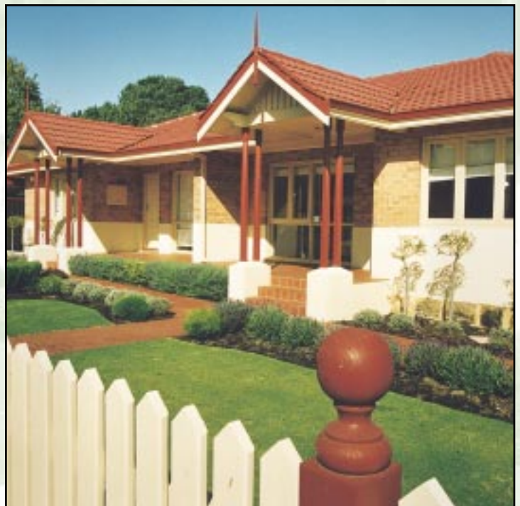
Refurbished Coolbellup property
