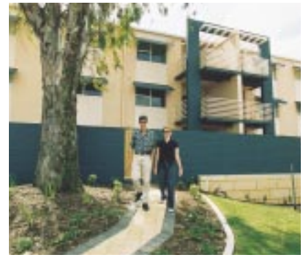
Ministry of Housing flats in Medina
