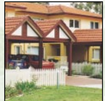
Refurbished townhouses in Lockridge
