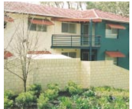
Medina flats after refurbishment
