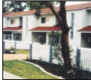
Refurbished Koondoola townhouses
