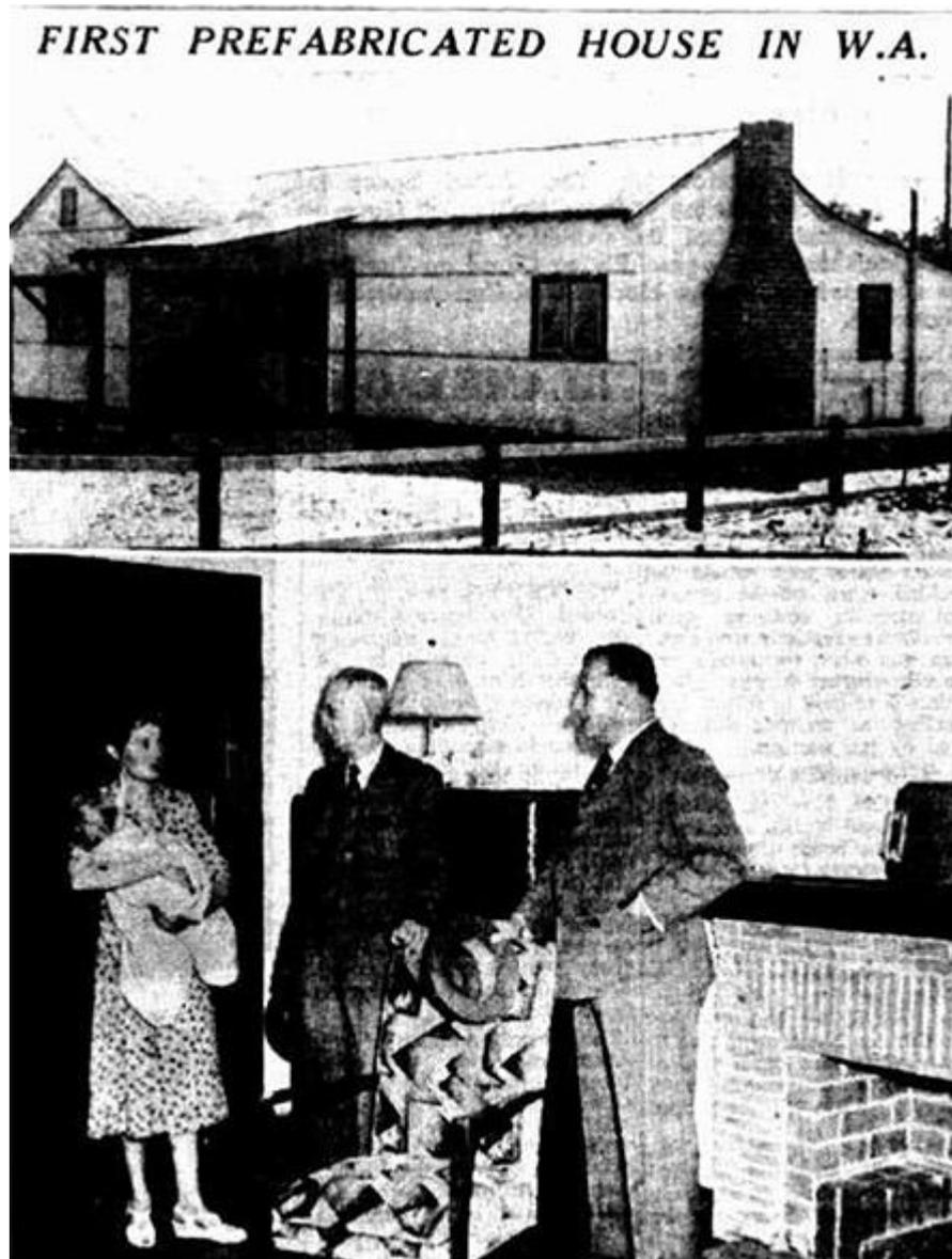
*The first prefabricated home built in Western Australia. Situated in Welshpool, the house had a timber frame and asbestos outside*
